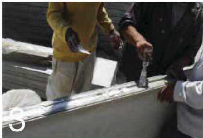
Apply adhesive to the mating surfaces and slide the next panel into position
