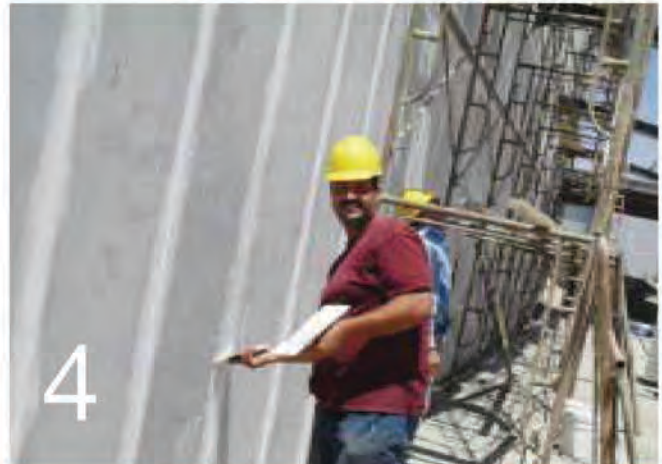
Tape LW-Panel joints and fill
