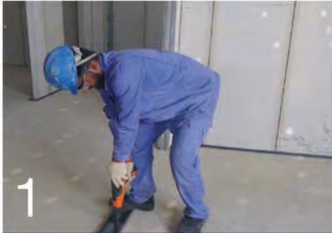
Fix U Channels to floor and ceiling/beam
