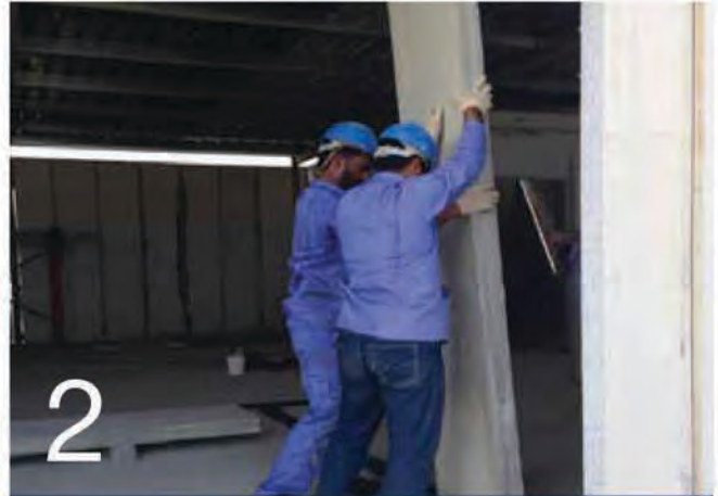
Place the panel in the channel and slide into position
